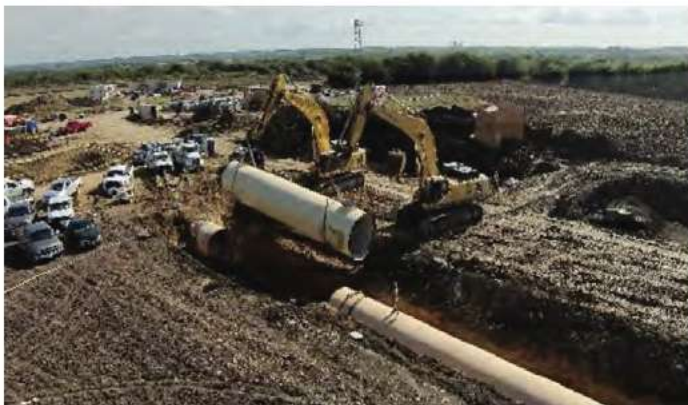
Section 12-13-MBR – Installation of 108-inch welded steel pipeline
