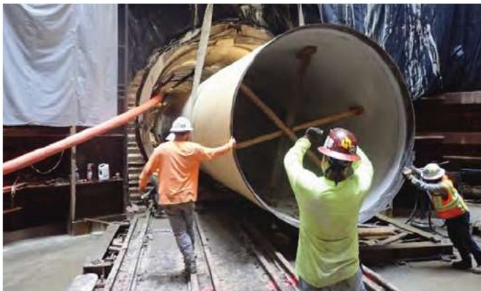
Section 17 Trinity Tunnel – Installation of 108-inch steel pipe in tunnel
