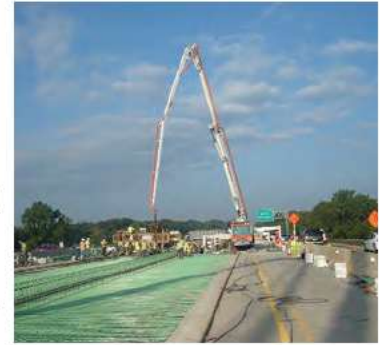
I-80 Roadway Construction
