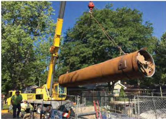
Jared Hamilton oversaw the auguring of dual 24-inch DIP water main 20 feet below the Eden's Expressway for MGNWC.
