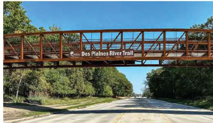
FPDCC Des Plaines River Trail Improvement Project
