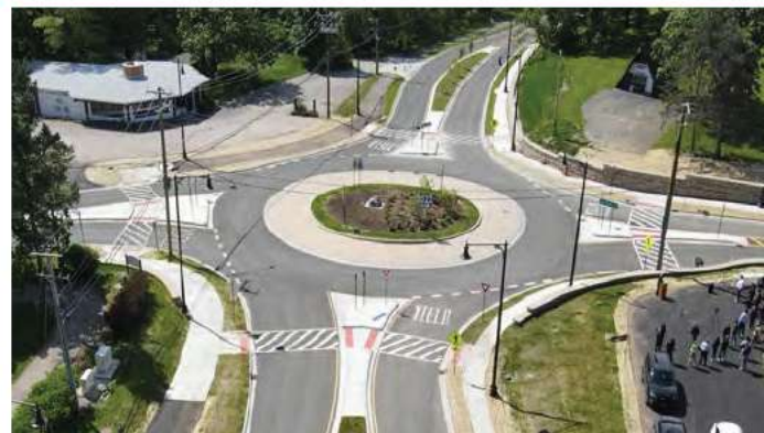
Algonquin Main Street Reconstruction Project
