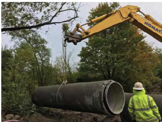
Established and effective construction management activities
