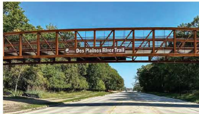
FPDCC Des Plaines River Trail Improvement Project
