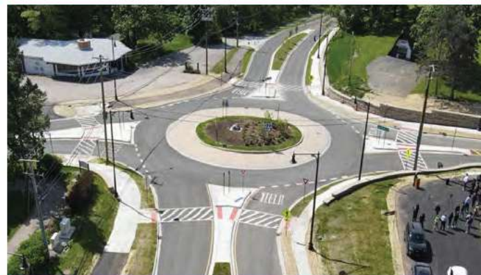
Algonquin Main Street Reconstruction Project
