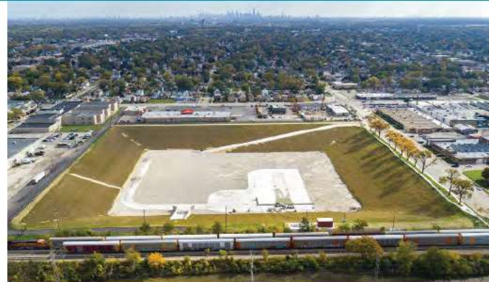
MWRDGC Addison Creek Reservoir Project
