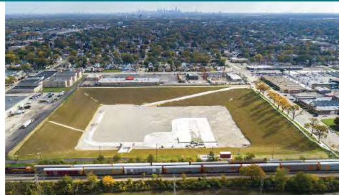
MWRDGC Addison Creek Reservoir Project
