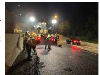
I-90 Night Construction 289 of 420
